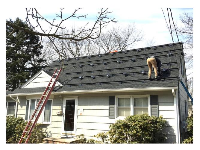
New GAF HDZ Roof Replacement Shingles Installed New Sunpower Solar System being installed on new GAF roof
